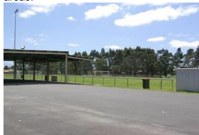
Extensive covered area from pavilion to side of soccer pitch.
