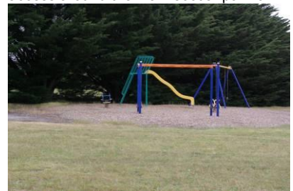
Children's Playground – very limited with equipment and isolated away from oval, tennis courts and soccer fields. Has potential CPTED risk issues with the close proximity of the large Cyprus pine hedge.
