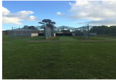
3 Practice Nets with synthetic grass with chain wire fencing. Wickets aged and in need of replacement
