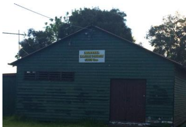
Pigeon Club building. Aged facility needing refurbishment
