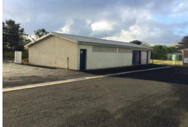
Cricket store room within the car park area. Aged facility
