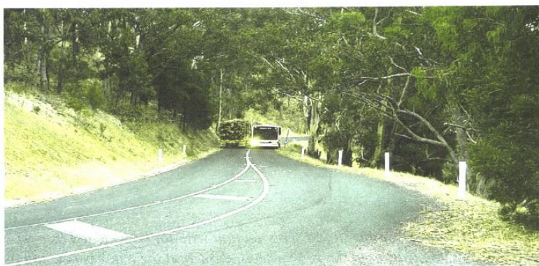
The log truck had to put its wheels in the unsealed gutter to squeeze past the school bus. A rear wheel of the bus is on the narrow, unstable verge beside a drop-off. (Jumbuk Road, just below Roberts' corner)
