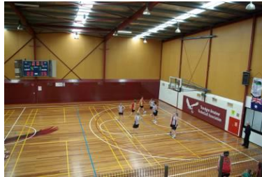
Courts multi-line not clear. Also safety run-off for both netball and basketball not to sports specifications (3.05m for netball & 2.0m for basketball).
