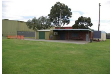
Overall the sports pavilion is in a fair condition
