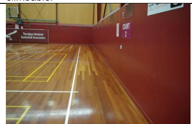
Safety run-off for both netball and basketball not to sports specifications along the sides of the courts as well as the ends (3.05m for netball & 2.0m for basketball).
