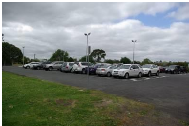
Main car parking in a fair condition – no apparent kerbing or storm water collection. Accessible car spaces are at distance from main entry.
