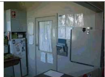
Image 6: Access door (egress doors) from maternal and child health rooms into the pre-school staff kitchen. Door shouldn't be considered as an egress door as this door will obstruct access from the pre-school side and the current door hardware is not compliant to BCA regulations as it can be lockable.
