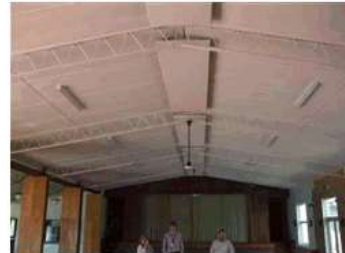
Image 9: Main ceiling in a reasonable condition.
