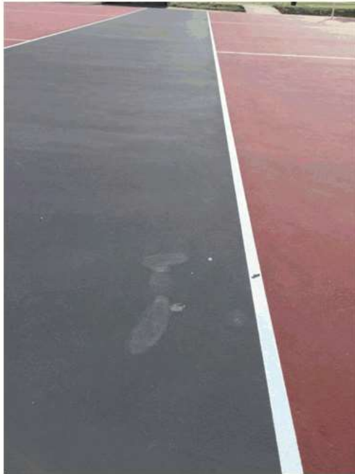
Delaminated acrylic area between Courts 6&7 with a piece of delaminated acrylic sitting freely on the court surface.
