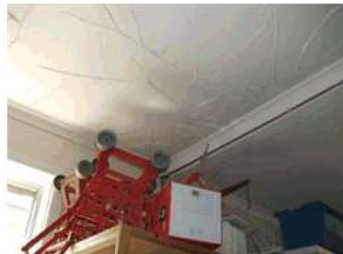
Image 10: Main store room – location of some equipment not readily accessible and issues with working at height to store equipment. Store room may require a better storage solution or more room. Water damage apparent to ceiling lining.
