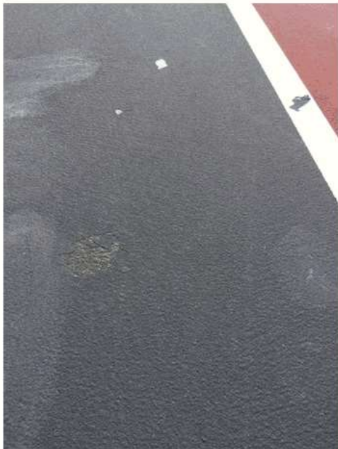
Close up of delaminated acrylic area between Courts 6&7 shows the glossy Qualipur Primer underneath.
