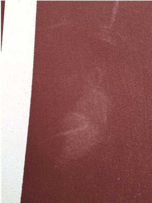
Example of faded acrylic colour where light scuffing has occurred. Sand is sitting freely on the surface.
