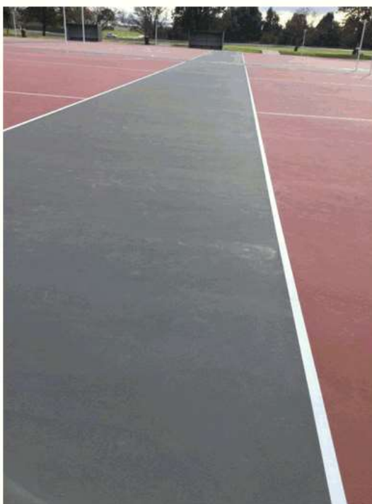
Patched area between Courts 9&10.
