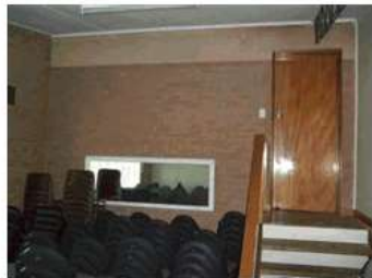
Image 10: Main stage is only accessible via steps. Height of stage is over 600mm – it may require barricades while not being utilised.
