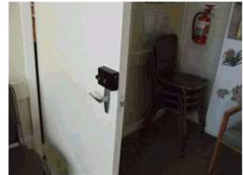
Image 6: Access door (egress doors) from maternal and child health rooms into the pre-school staff kitchen. Door shouldn't be considered as an egress door as this door will obstruct access from the pre-school side and the current door hardware is not compliant to BCA regulations as it can be lockable.
