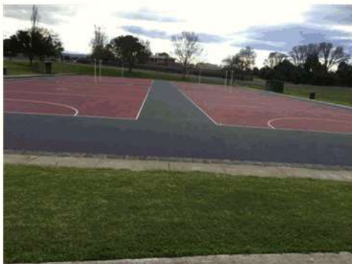
View of the Courts 1-4 pavement area, looking North.
