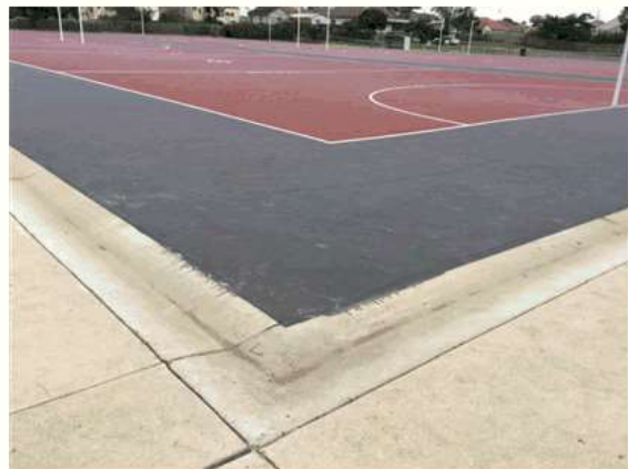
Excess Qualipur Poly Primer on concrete spoon drains.
