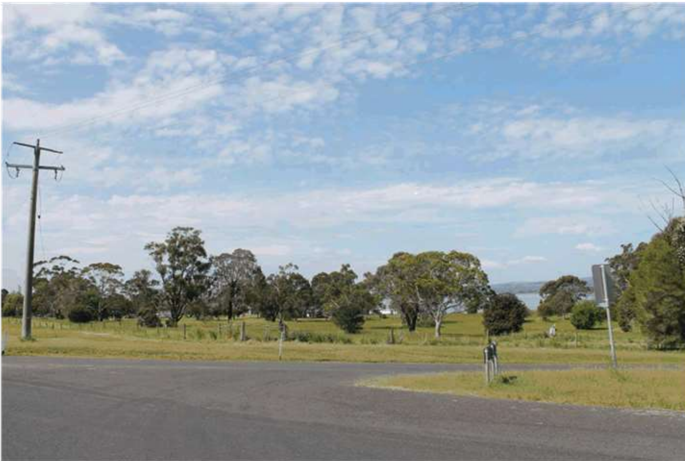
Existing site from Yinnar Road
