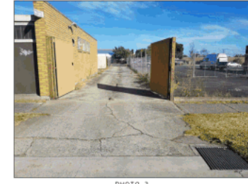
PHOTO 3 LOOKING WEST DOWN EXISTING LANEWAY (FROM COLLINS STREET)
