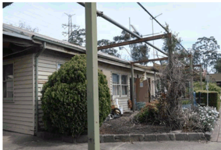
Technical training centre (southern section)
