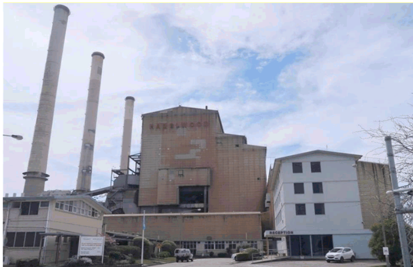
Hazelwood Power Station, 2018
