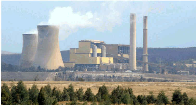
Yallourn W Power Station
