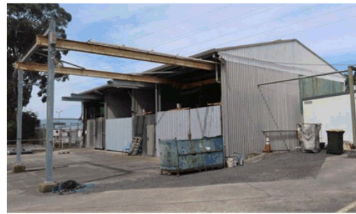
Boiler tube store (former hydrogen production plant)
