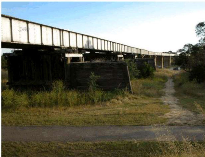
The existing Avon River bridge at Stratford
