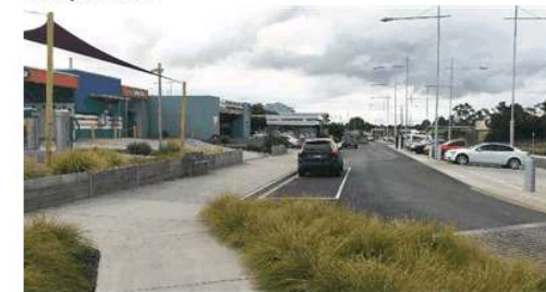
Figure 3 – Existing Commercial area accessed via Philip Parade
