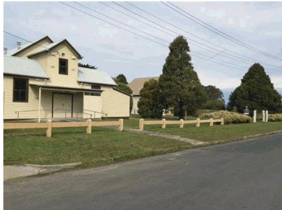
PHOTO 7 – Mechanics Institute Hall, St Johns Anglican Church and residential development in Railway Avenue
