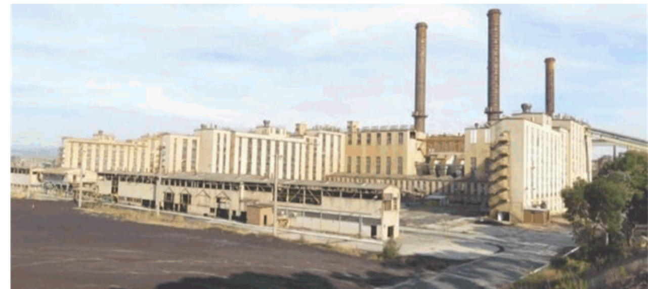
The Morwell Power Station and Briquette Factories Victorian Heritage Database
