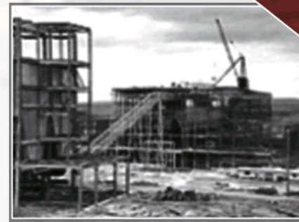
Construction of Power Station and Briquette factory Morwell, November 1956 Museums Victoria
