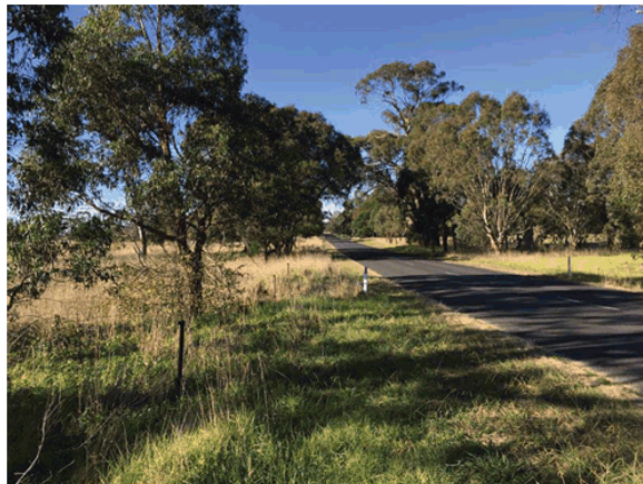
PHOTO 2 – Cairnbrook Road adjacent to the site, facing east
