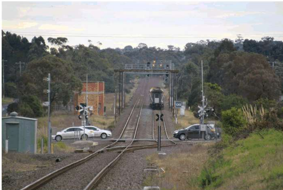
Bunyip – looking towards Melbourne Trains diverging from the single line to double lines and vice versa at Bunyip and Longwarry must slow to 65 km/h while passing through these points
