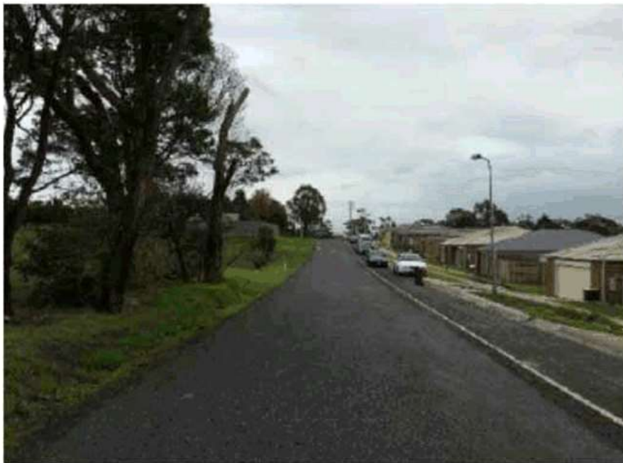
Figure 4 Glendonald Road looking west 4
