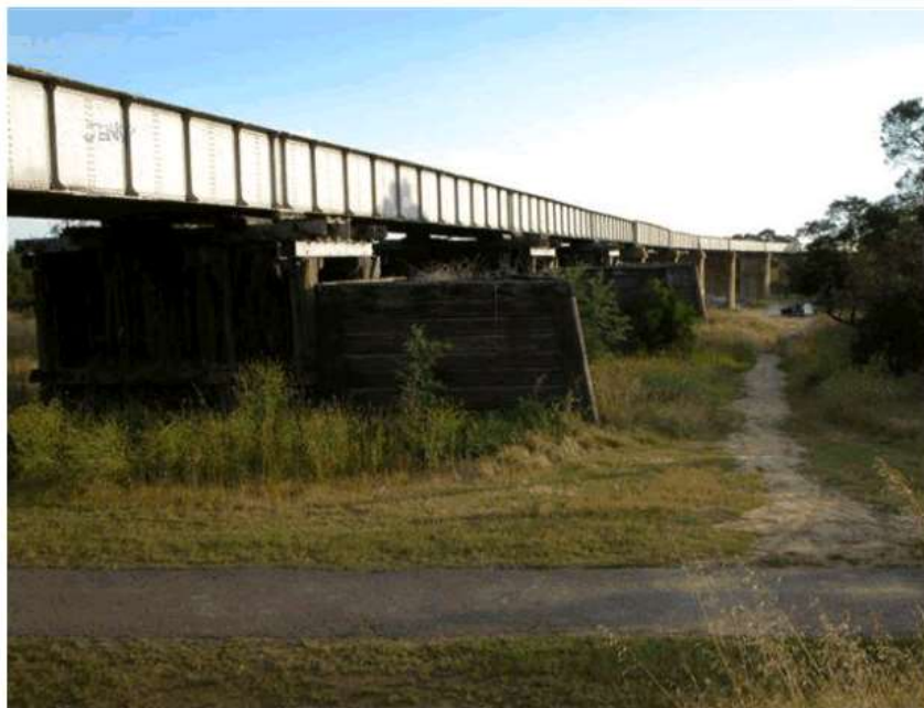
The existing Avon River bridge at Stratford
