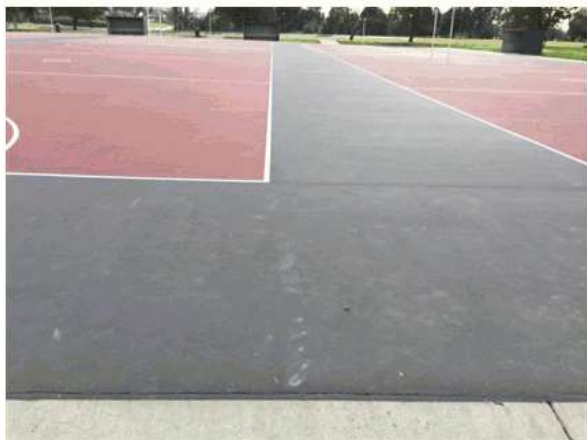
Previously repaired areas along the Southern boundary of Courts 5-10.
