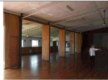
Image 6: Main hall showing operable walls between main hall and supper room.
