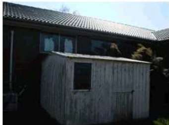
Image 10: Old metal clad store room located within southern garden space.
