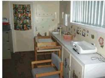
Image 4: Staff kitchen area restricted. No evidence of hands free basin for food prep. Only door accessing the southern garden area. This door shouldn't be considered an egress door as there is no emergency access from the garden to a nominated emergency point outside the property. Note – existing exit sign not compliant. Requires to be illuminated. Door hardware not compliant.
