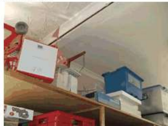
Image 11: Main store room – location of some equipment not readily accessible and issues with working at height to store equipment. Store room may require a better storage solution or more room.
