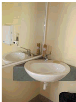
Image 2: Basin appears in the wrong position relating to pan and mirror.
