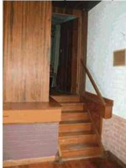
Image 10: Main stage is only accessible via steps. Height of stage is over 600mm – it may require barricades while not being utilised.
