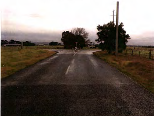
Figure 2.7: Park Lane (North of Mayfair Court) Looking North
