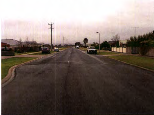
Figure 2.9: Park Lane (South of Mayfair Court) Looking North
