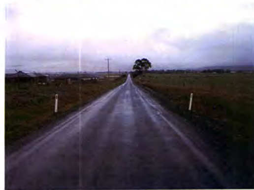
Figure 2.4: Marshalls Road Looking West
