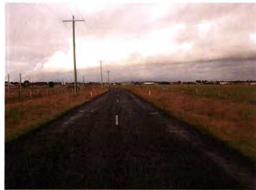
Figure 2.8: Park Lane (North of Mayfair Court) Looking South
