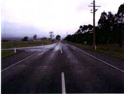
Figure 2.5: Traralgon – Maffra Road Looking North
