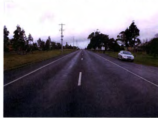
Figure 2.6: Traralgon – Maffra Road Looking South
