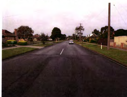
Figure 2.14: Morgan Drive Looking West
