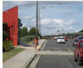
Existing entrance and footpath along Latrobe Leisure Centre
