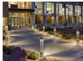
Example of well defined entrance
