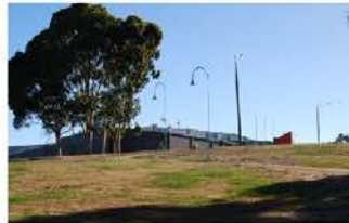
Existing embankment - between Eel Hole Creek and Latrobe Leisure Centre, view towards Leisure Centre
