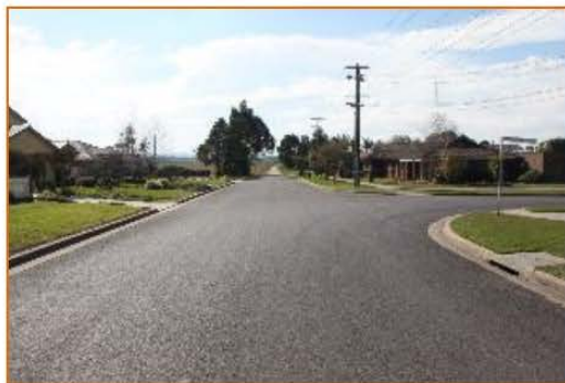
Figure 3 Catherine Street Facing North from Adjacent Bellarine Circuit
