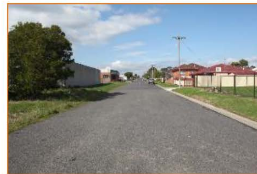
Figure 7 Mary Street Facing East Towards Davey Street
