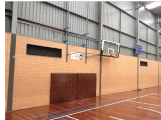
Not enough padding to goal end of courts 2 + 3. Padding should extend the length of the goal zone for netball and not just cater for the basketball key. Also not enough safety run off for both basketball (2.0m) and netball (3.05m)
