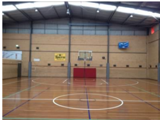
Stadium 1 - Not enough padding to goal end of courts 1. Padding should extend the length of the goal zone for netball and not just cater for the basketball key. Also not enough safety run off for both basketball (2.0m) and netball (3.05m) at goal ends.
