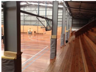
Safety run-off zone between courts, columns and seating too narrow. Pedestrian gap between seating and columns non-existent. Padding to wrap around columns and not just playing side.
