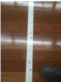
Stadium 1 - Nails protruding from main sports floor in Court 1. Not safe. Should be rectified immediately.
