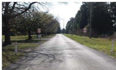
Photo 5 - Looking along Toners Lane
