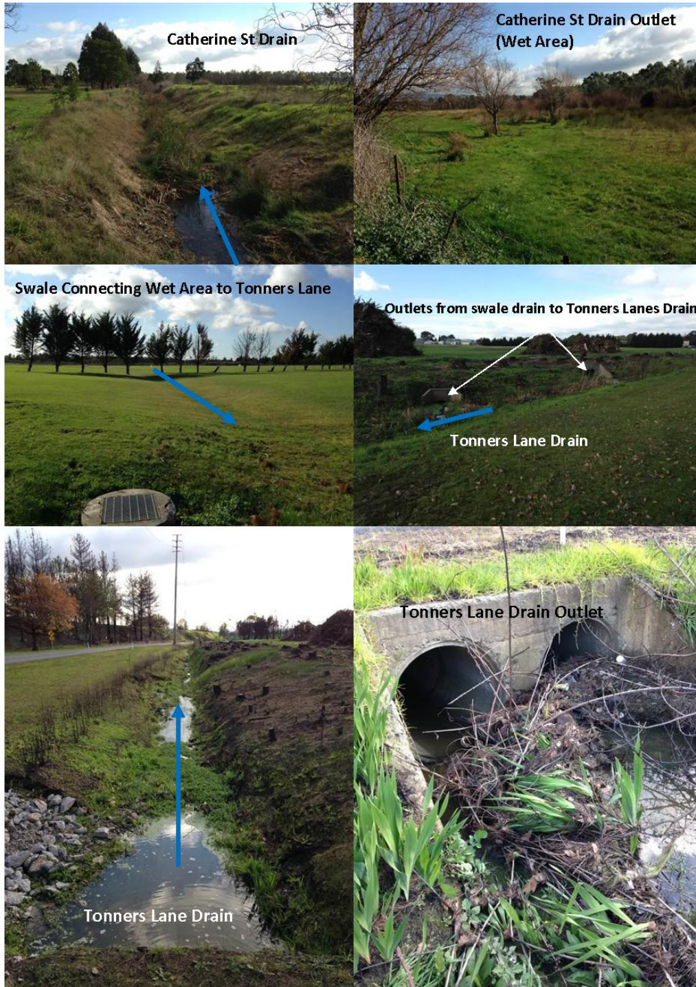
Figure 2-3 Site Visit images
