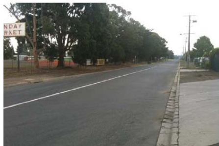
Photo 4 - Looking along Latrobe Road
