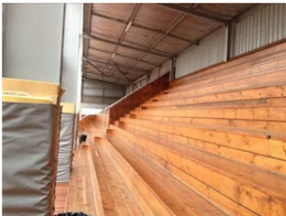
Timber tiered seating – too steep. May be considered not compliant to current BCA & DDA regulations.
