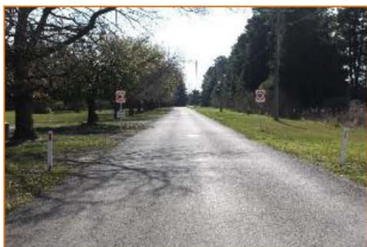
Figure 8 Toners Lane Facing North Adjacent the Subject Site
