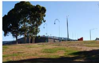
Existing embankment - between Eel Hole Creek and Latrobe Leisure Centre, view towards Leisure Centre
