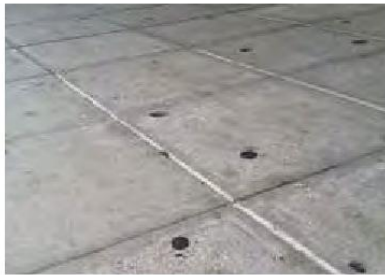
JOINTED CONCRETE PATH
