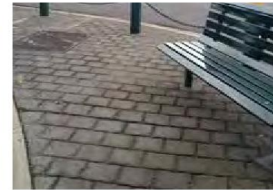
CONCRETE STENCILLING AND PRESSING
