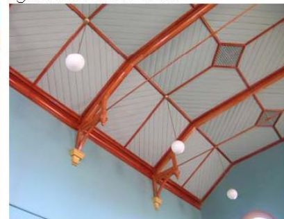
Figure 3.25 Court Room ceiling
