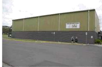
Existing stadium (southern courts) appears in a reasonable condition. Evidence of wear and tear at close inspection.
