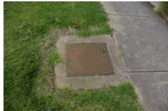
Site is restricted along boundaries with service authority easements. All easements will need to be located including in ground services before any redevelopment works are to proceed.
