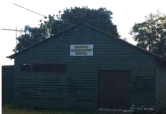
Pigeon Club building. Aged facility needing refurbishment
