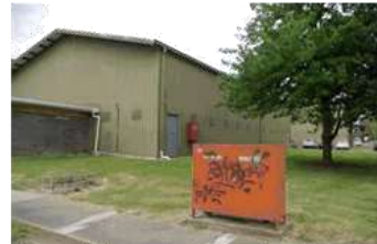
External fire services ‘may’ require upgrading as part of any sports reserve redevelopment.
