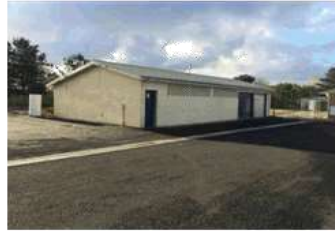
Cricket store room within the car park area. Aged facility
