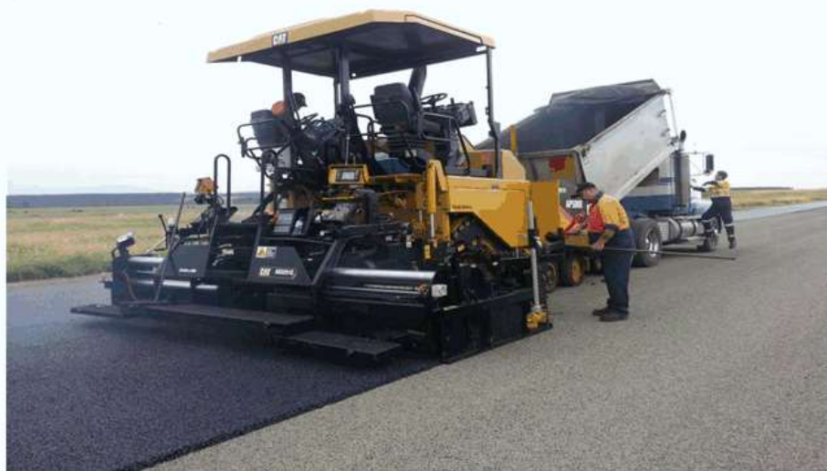
Resurfacing the Main Runway (see also front cover photo)
