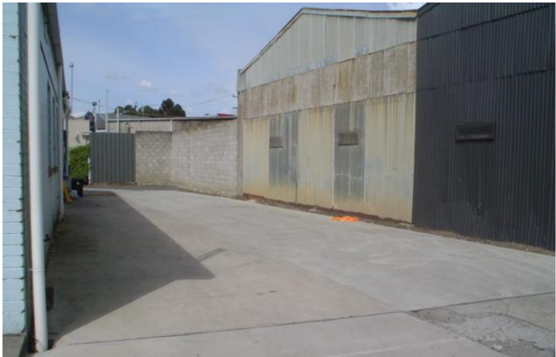
Close up of Lane Entrance
