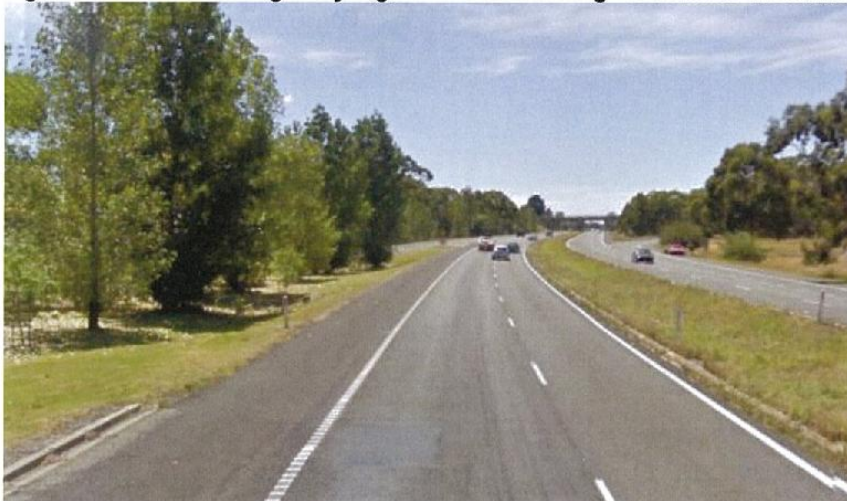
Figure 2: Trees blocking early sight lines of entering vehicles to the Princes Highway
