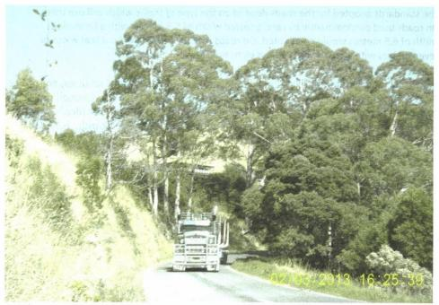
This is a typical section of Jumbuk Road. This section will not be widened as part of the programmed works. The position of the rear wheels show that the truck is keeping as far to the left as possible. If an oncoming vehicle met this truck on the bend behind the truck, the vehicles would have nowhere to go and no time to stop.
