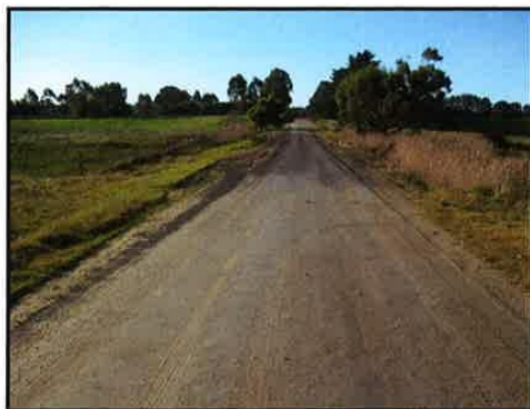
Photograph 5: Silcocks Road (North-South Leg) - View North
