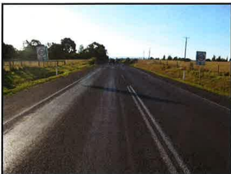
Photograph 3: Monash Way - View North
