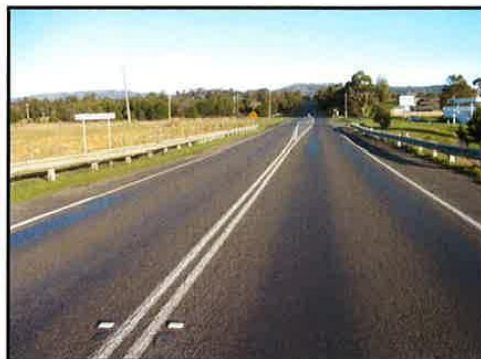
Photograph 4: Monash Way - View South
