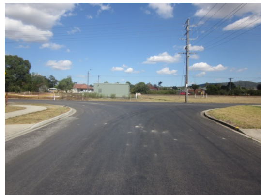
Figure 2.9: Mitchells Road (Waterloo Road intersection facing South)
