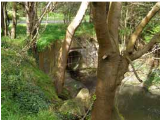
Photos 3 and 4 Mitchells Road Drain pipeline (1500 mm diameter) at outlet to open waterway 100 m south of Saviges Road and at inlet to pipeline under Mitchells Road
