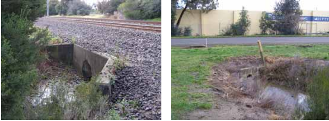
Photos 5 and 6 Culverts under Railway and Waterloo Road at Rocklea Mills
