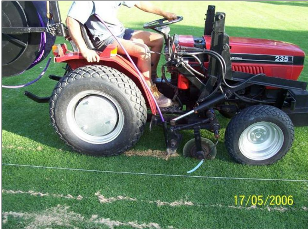
Figure 3. Photo of typical subsurface irrigation installation from Netafim brochure. Note the cutter wheel making a narrow slot for the pipe that rolls off the drum and is inserted below the surface.
