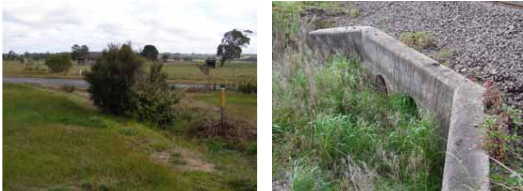
Photos 11 and 12 Culverts under Railway and Waterloo Road at Old Gippstown Drive alignment. Part of Area 3 is downstream of Waterloo Road.
