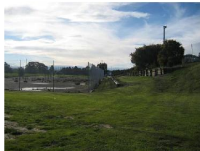
Figure 22: Embankment west of tennis courts
