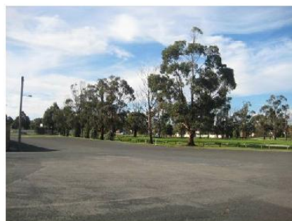
Figure 19: Main car park
