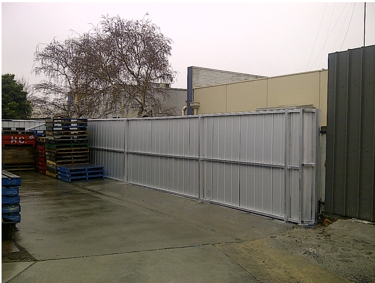
Permanent Fence Erected July 2013
