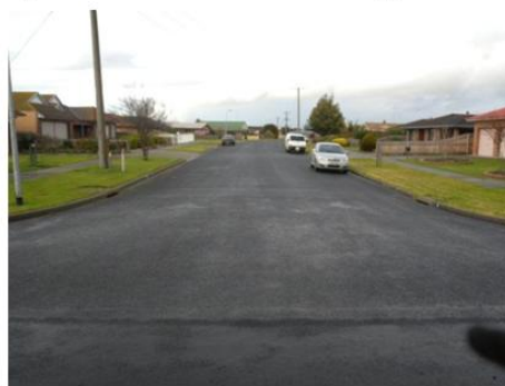
Figure 2.12: Greenfield Drive Looking South
