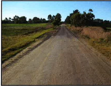
Photograph 5: Silcocks Road (North-South Leg) - View North
