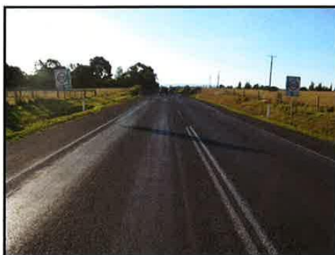
Photograph 3: Monash Way - View North
