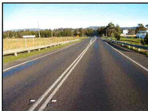
Photograph 4: Monash Way - View South
