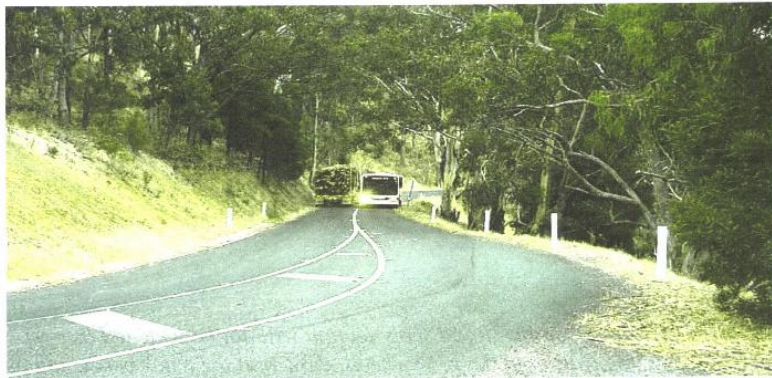
The log truck had to put its wheels in the unsealed gutter to squeeze past the school bus. A rear wheel of the bus is on the narrow, unstable verge beside a drop-off. (Jumbuk Road, just below Roberts' corner)
