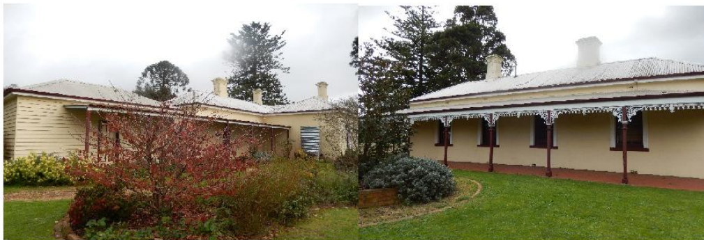
Homestead Eastern View
