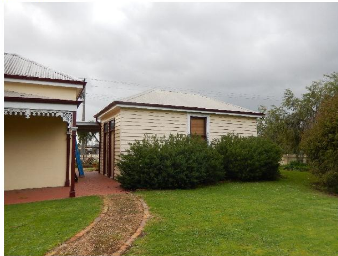
Western View of Meeting Room and Toilets
