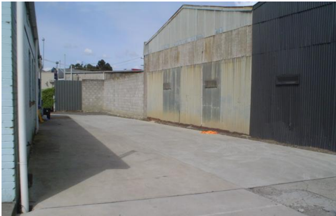
Close up of Lane Entrance
