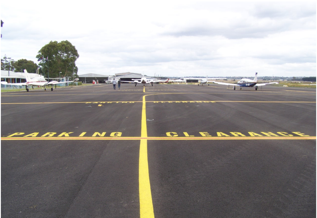
(Pictured above – Main Apron Area Refurbishment)
