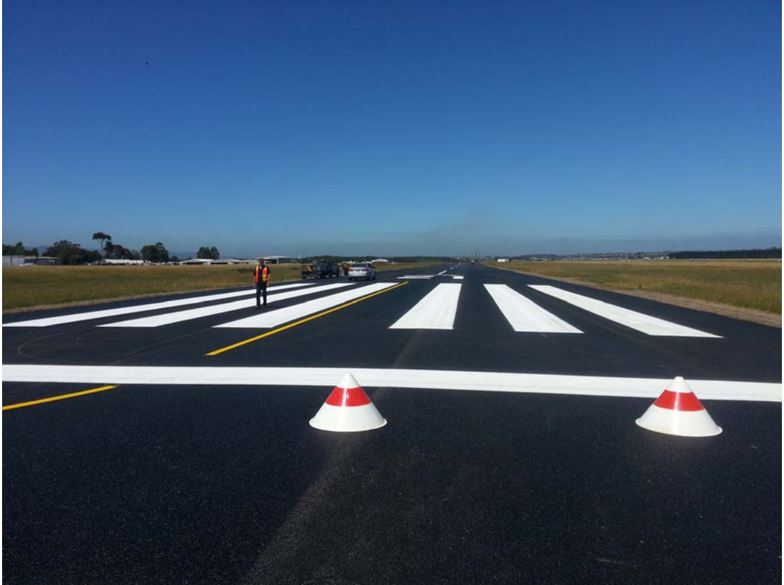
(Pictured above: Sealing of the main runway 03/21)
