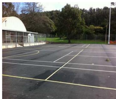
Figure 17: Multi use courts constructed at Boolarra
