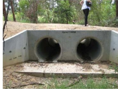
Figure 15: Drain beneath North Boundary Track
