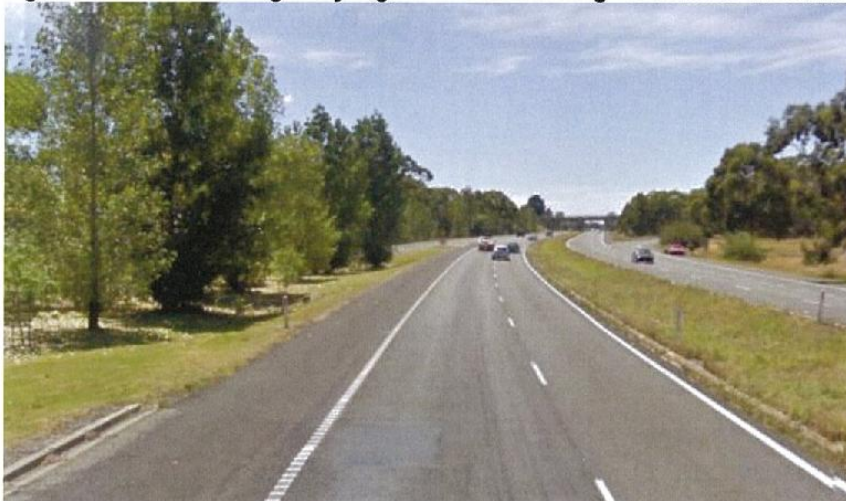
Figure 2: Trees blocking early sight lines of entering vehicles to the Princes Highway
