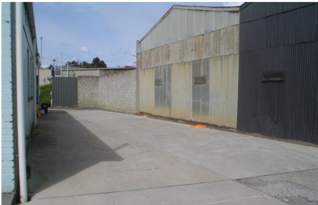
Close up of Lane Entrance
