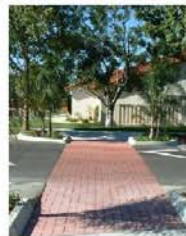
Example of raised pedestrian crossing
