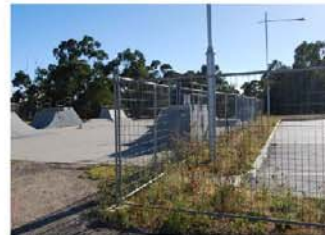
Existing interface between skate park and car park
