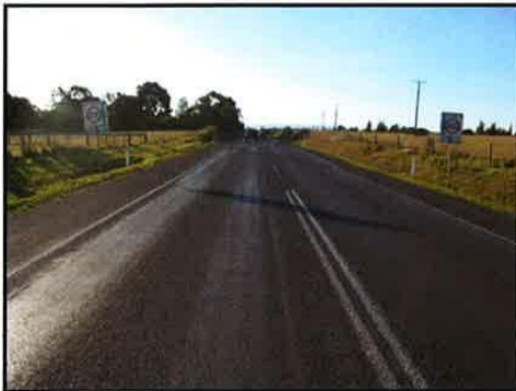
Photograph 3: Monash Way - View North
