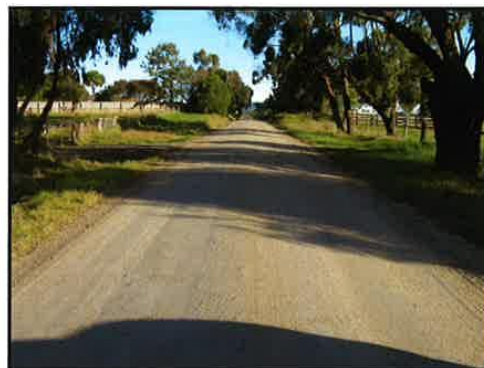
Photograph 6: Silcocks Road (North-South Leg) - View South
