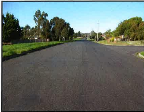
Photograph 1: Acacia Way - View East
