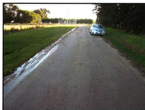
Photograph 8: Silcocks Road (East-West Leg) - View West
