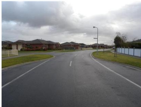
Figure 2.9: Franklin Street Looking East
