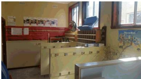
Existing coat rack area to be removed
