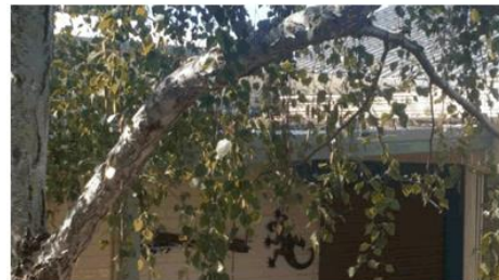
Entry area gutters
