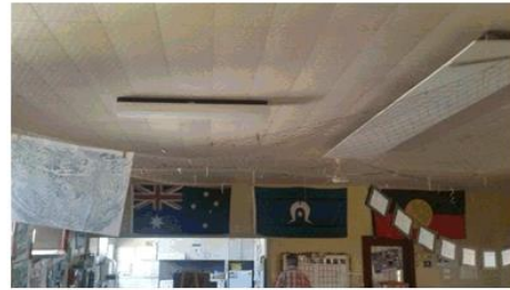
Pre-School main area
