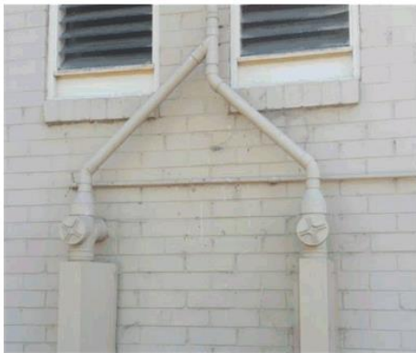
Sewer from Toilets at Stage to be removed
