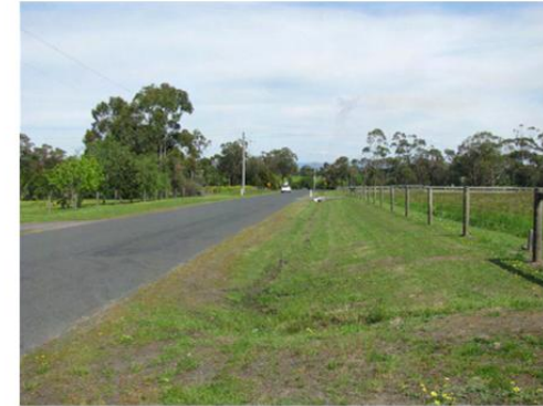
Image 16: View along road frontage
