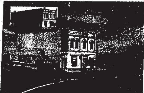
The Cobbedick building which was on the corner of Franklin St and the Princes Hwy.
