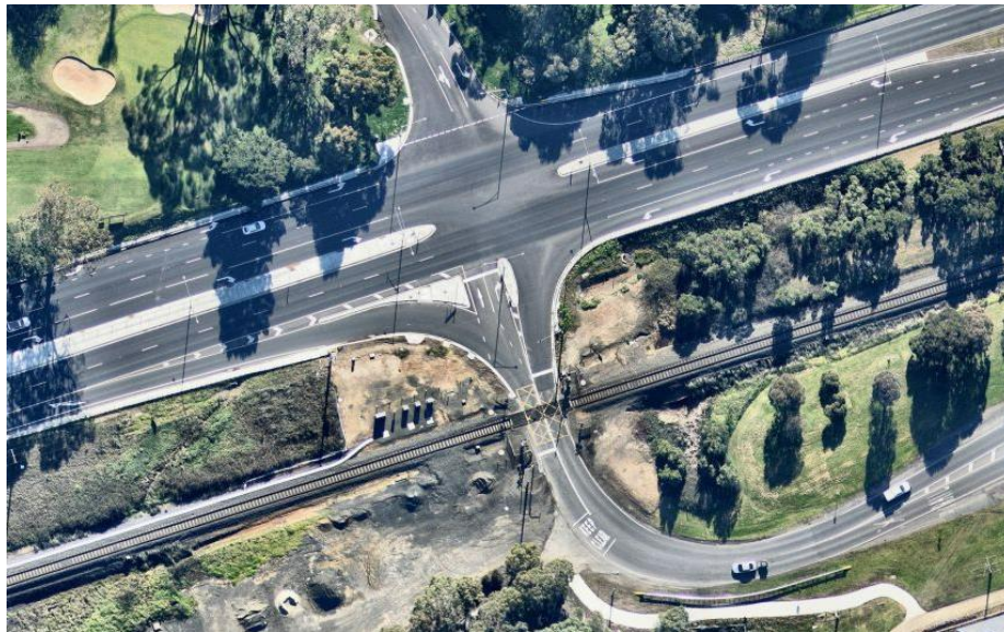
FIGURE 5 INTERSECTION OF PRINCES HIGHWAY AND BANK STREET AFTER THE RECONSTRUCTION
