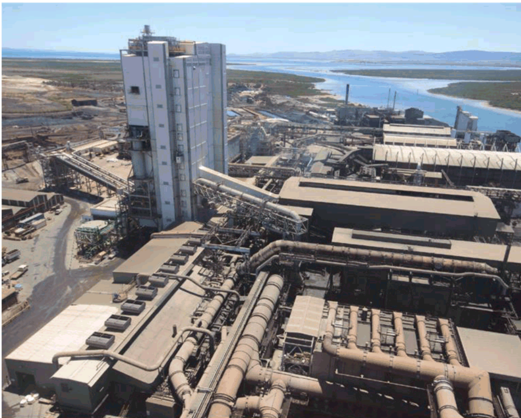
Figure 1 – Photograph of a part of the Port Pirie lead smelter (source unknown).
