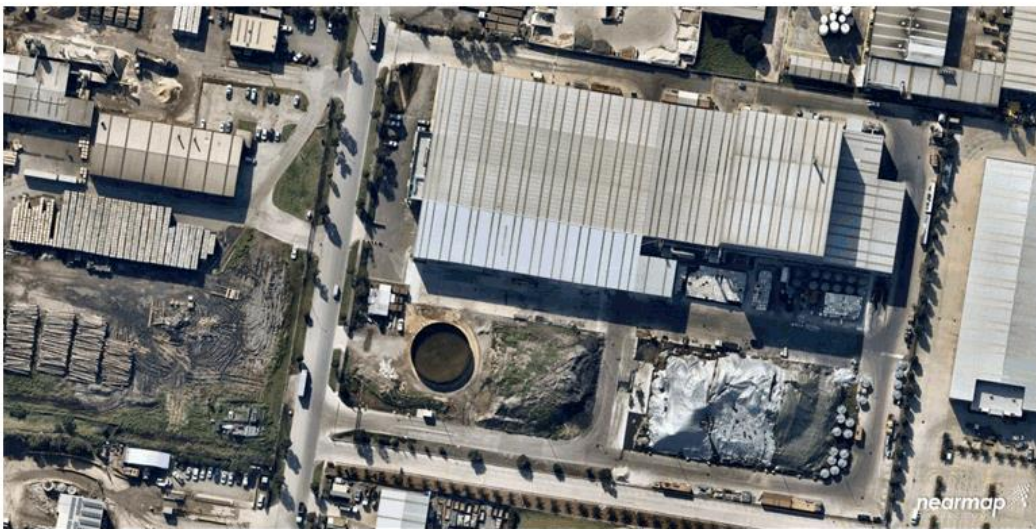
Figure 4 – Renex Facility – 2020 showing more recent site developments and apparent storage of what is presumed to be treated soil in an external, covered stockpile (Image from NearMap).
