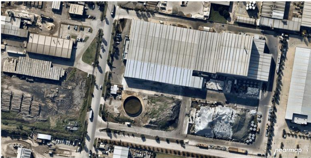
Figure 4 – Renex Facility – 2020 showing more recent site developments and apparent storage of what is presumed to be treated soil in an external, covered stockpile (Image from NearMap).
