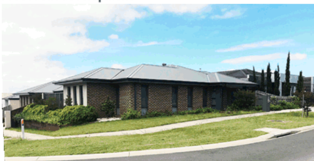
Example of a good quality corner dual occupancy development
