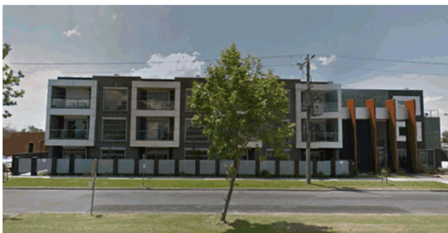
View of existing apartment typology in Traralgon
