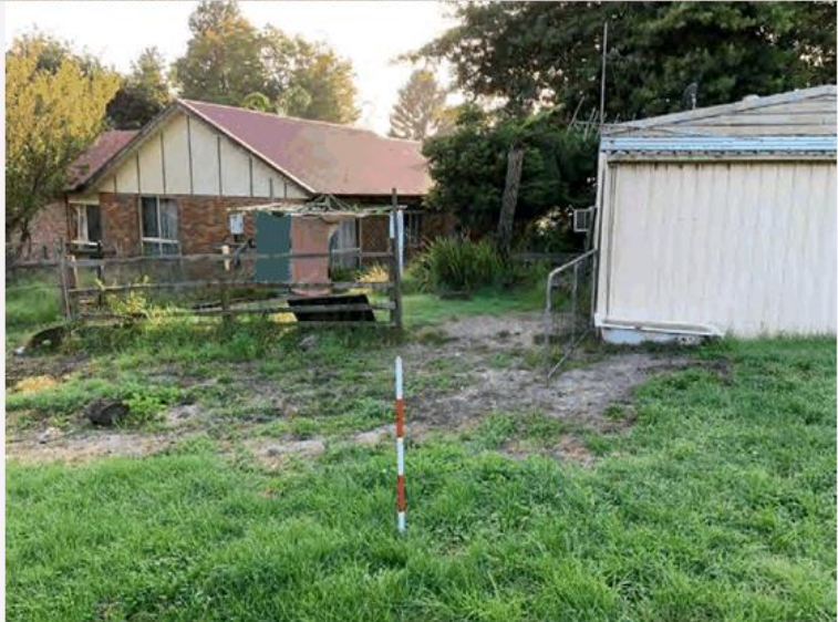
Plate 2: View of house, shedding and exposed grey silt (M. Barker 16/3/20), facing northwest.
