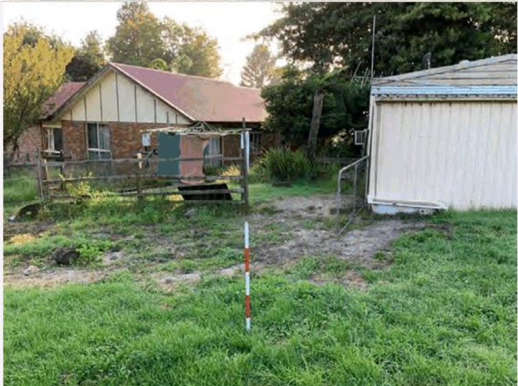
Plate 2: View of house, shedding and exposed grey silt (M. Barker 16/3/20), facing northwest.
