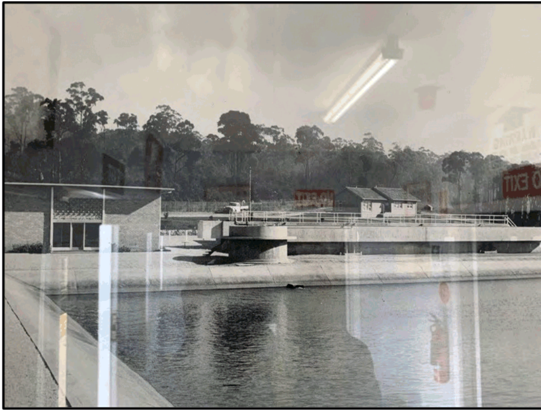
Figure 3: 1961 Photograph showing the Newly Constructed Treatment Plant with the Operators House at the Rear
