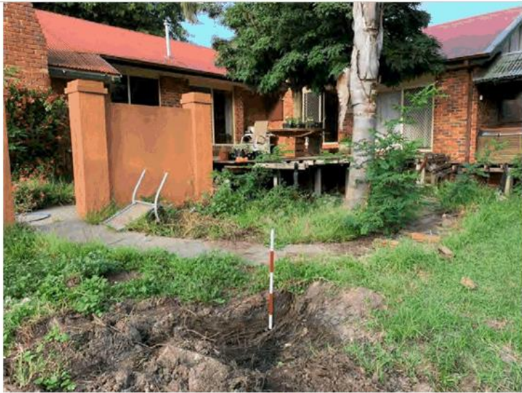
Plate 1: View of existing house on 58m Moe South Road (M. Barker 16/3/20), facing southeast
