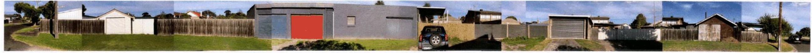
NO.22 NO.20 NO.18 NO.16 NO.14 FIGURE 1. BENTLEY STREET (LOOKING EAST)
