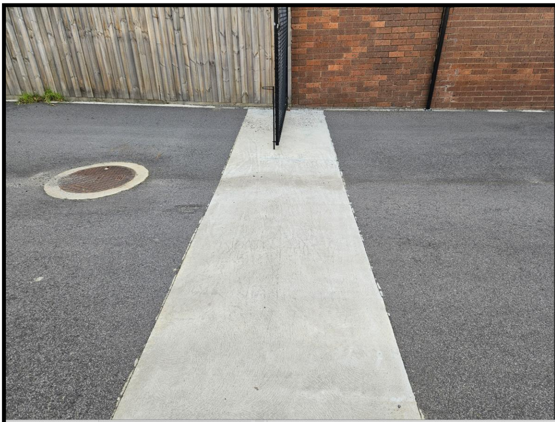
Reinforced concrete for gate construction
