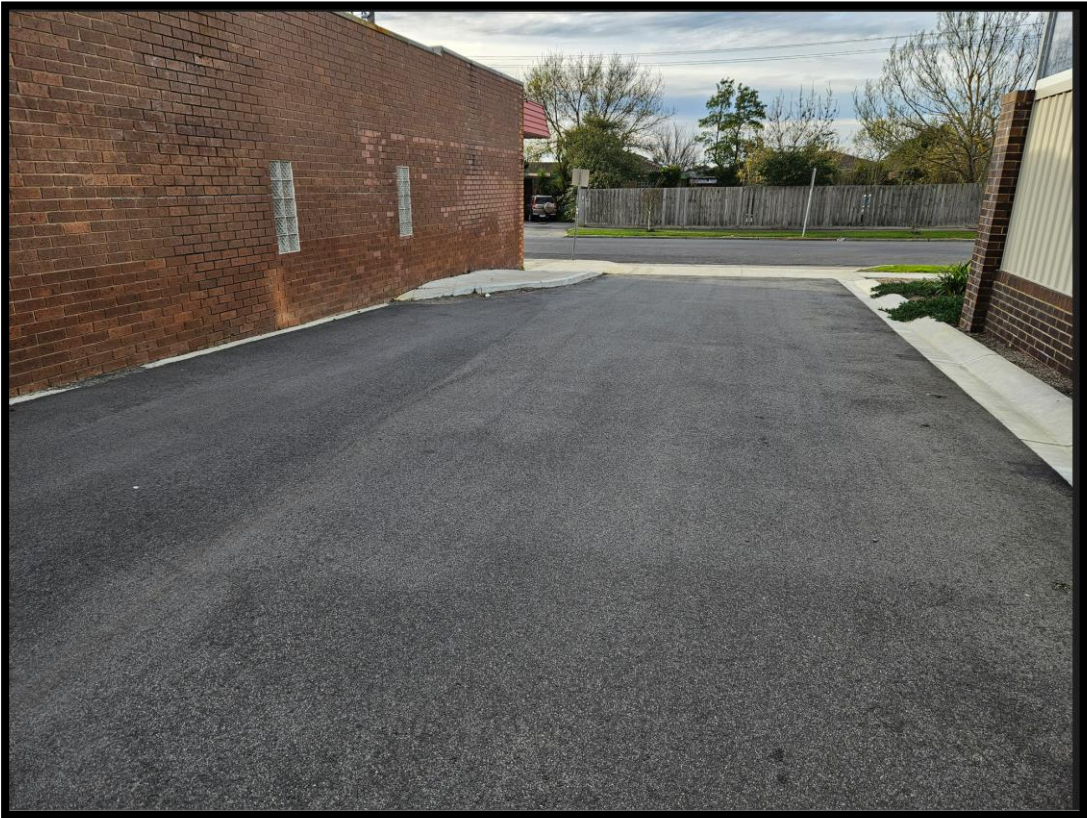
Construction of concrete island to steer vehicles in line with access
