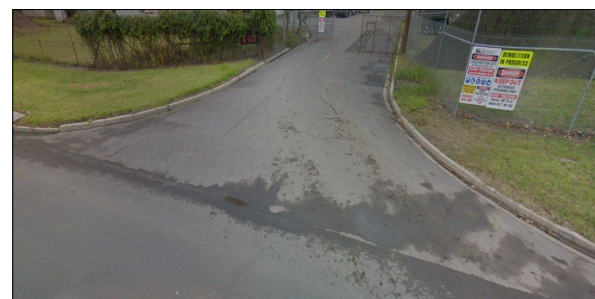
5 The existing vehicle crossing is conveniently located and is suitable for retention or to be upgraded as part of any development application.
